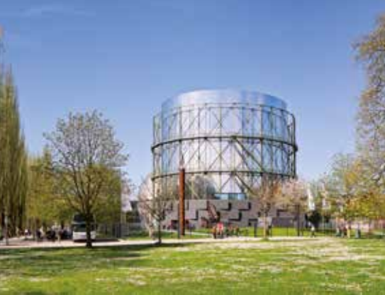
Gasometer in Pforzheim
